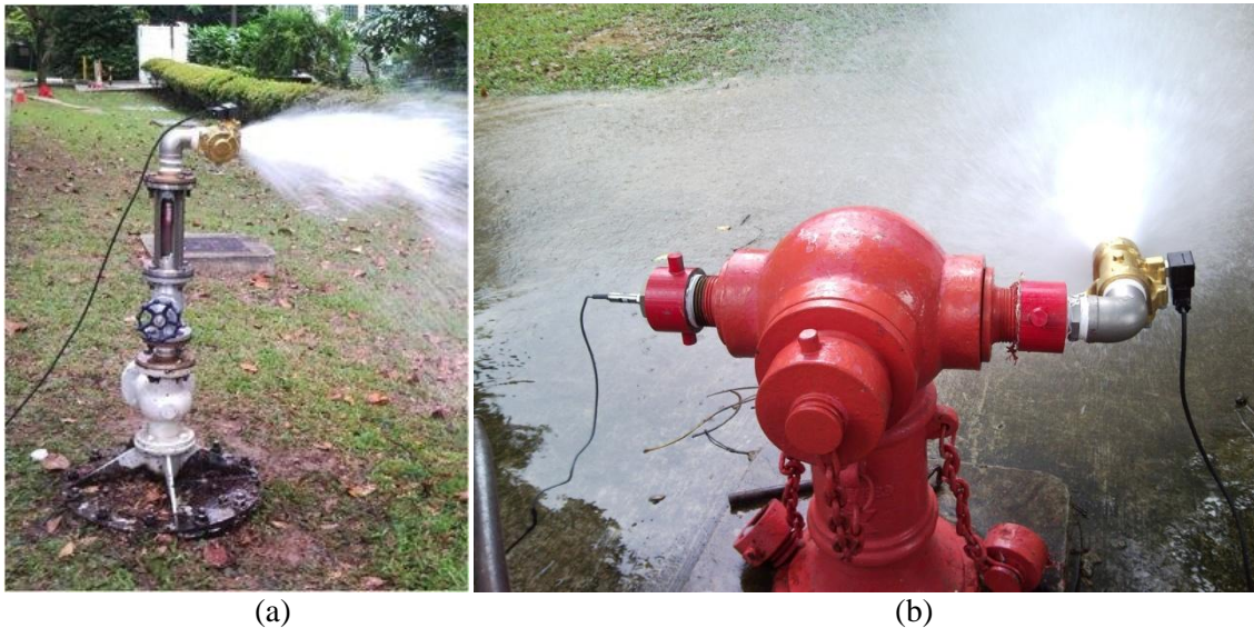
Figure 12. During leak-off experiments artificial bursts and leaks are generated by fast-opening solenoid valves connected to air valves (a) or fire hydrants (b)
